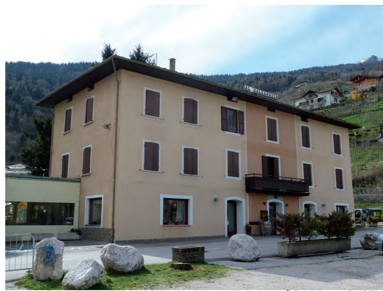
East view of the existing building
