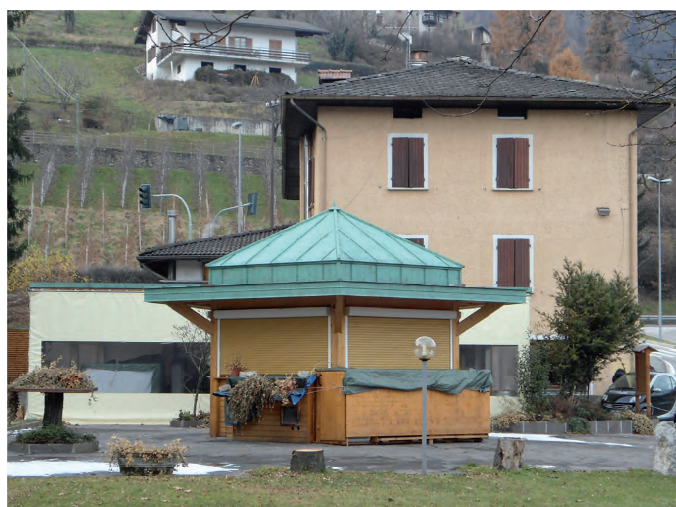
South - east view of the existing building
